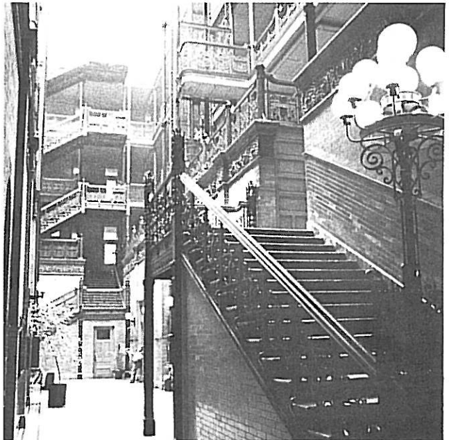
Interior, Bradbury Building
