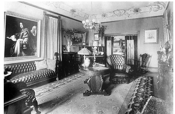
Parlor, pre-renovation. Photo: Glendale Public Library, Special Collections
