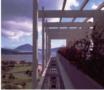
Kahala Hilton (1964) by Killingsworth. Photo: © J. Paul Getty Trust. Used with permission. Julius Shulman Photography Archive, Research Library at the Getty Research Institute
