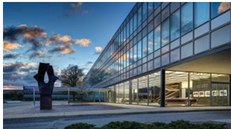
Styling (Design) Building, General Motors Technical Center, Warren (Eero Saarinen and Associates, 1956). Photo: James Haefner/Michigan State Historic Preservation Office
