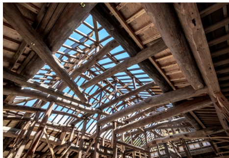
The original roof beams were used whenever feasible in the reconstructed framework of the house.
