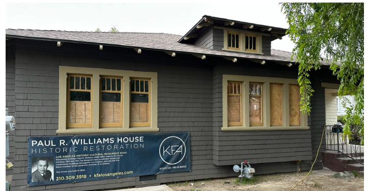
The 1905 bungalow in process of renovation by KFA Architecture.
